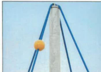
In the centre of the net is the mast, made of high quality seamless steel. The structure of the mast as an oscillating support is statically favourable and equalizes the oscillations in the net. The masts are hot dip galvanized as standard, with the design option of additional powder coating.
