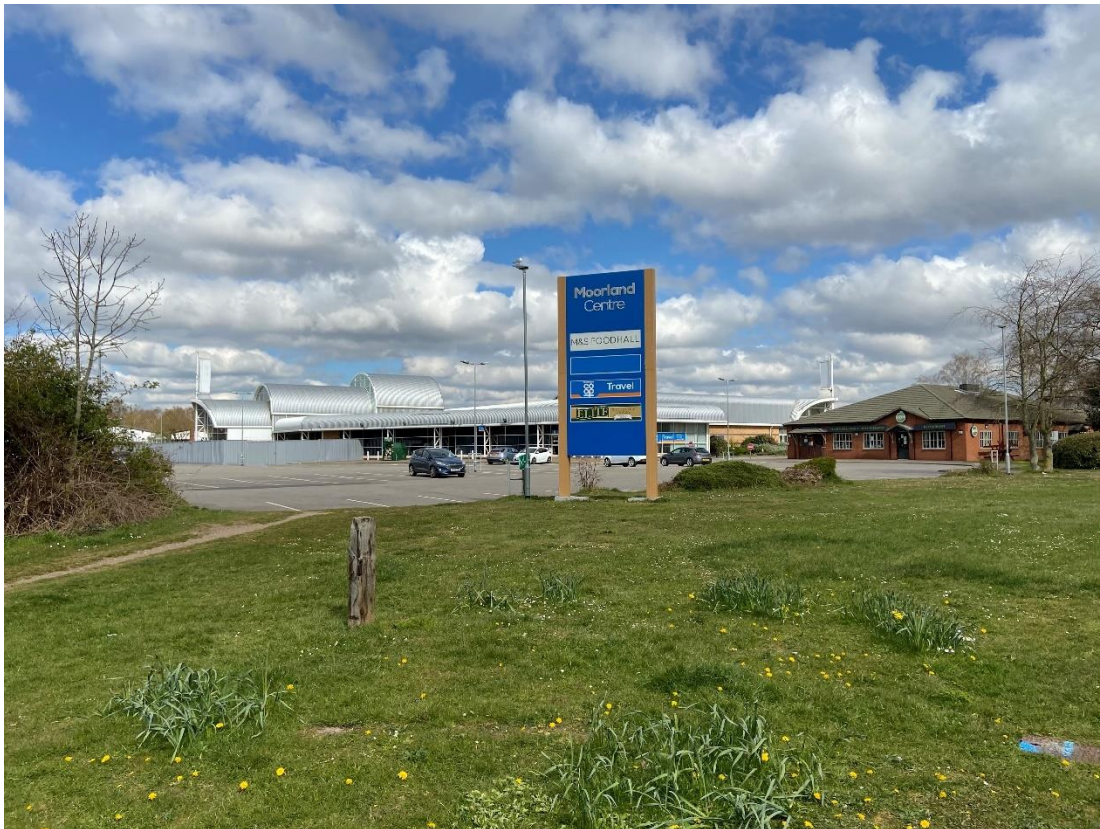
Existing Moorland Centre from Tritton Road with the Elite restaurant to the right
